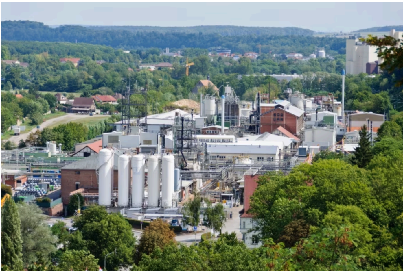
The Solvay plant in Bad Wimpfen, Germany, where TFA is still being used as a raw material and emitted into the Neckar river © Colin Utz/Alamy
